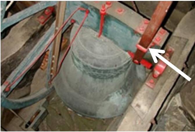
A plain stay on a wooden headstock, held on by 3 bolts (below) and a metal strap (above)
